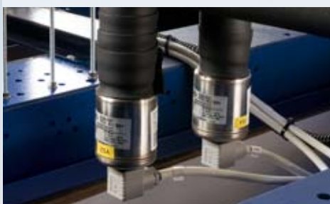
Electronic thermostatic expansion valves.
